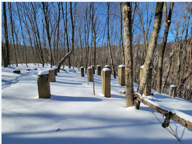
Pilings for the dance hall.
